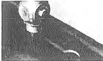
Cutting ductile iron pipe with abrasive wheel.
