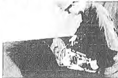
Cutting ductile iron pipe with abrasive wheel.
